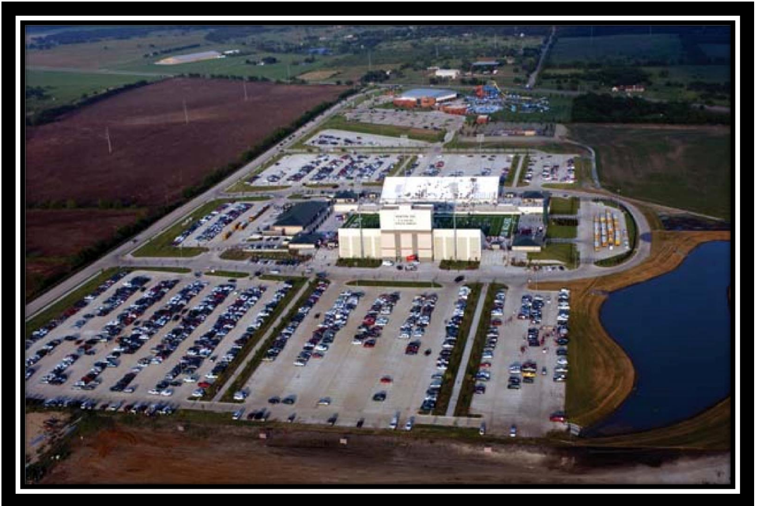
Aerial View of C.H. Collins Athletic Complex Denton Independent School District Denton, Texas
